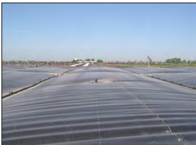
Anaerobic lagoon producing biogas from hog manure in California's San Joaquin Valley
