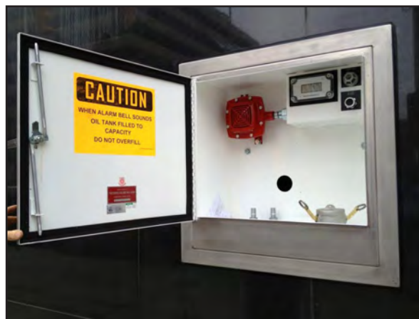
Interior view of an installed Model 2 fill box with Electronics Package No. 4 and a solenoid overfill prevention valve.
